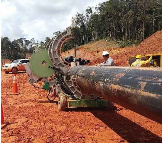
Fig.4: Fusion of 24-inch HDPE at Newmont
