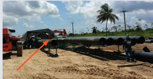
Fig.8: MEGAMC Polyhorse installation
