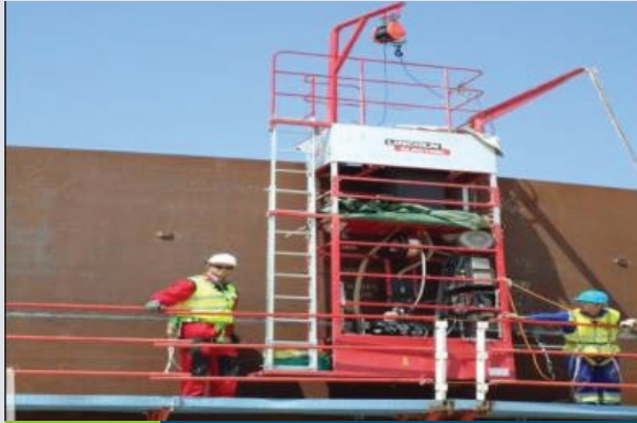
Fig.10b: Welding "robot" - Roof
