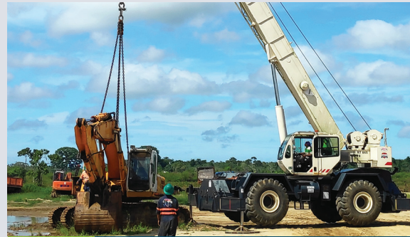
Fig.17: 65 Ton Terex mobile Crane
