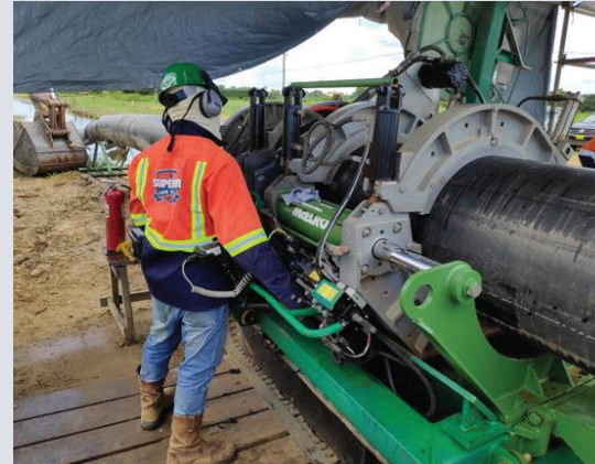
Fig.1: Fusion of 22-inch HDPE pipe
