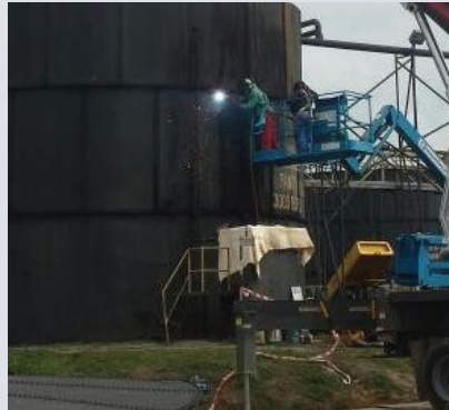
Fig.12a: Demolishing of tank (gouging)
