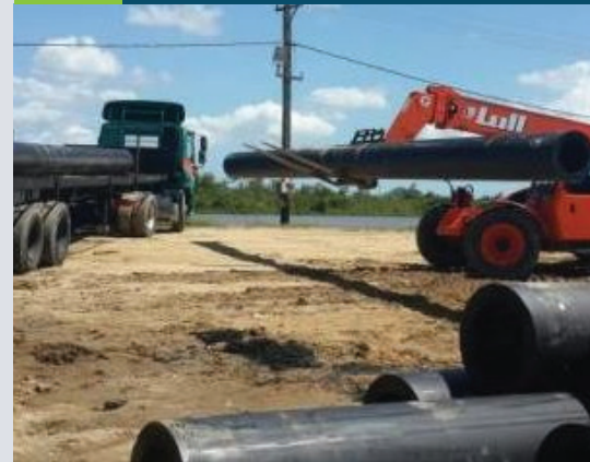
Fig.2: Pipe handling during fusion jobs
