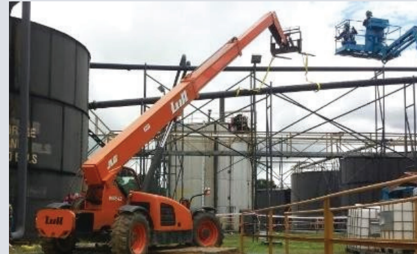
Fig.12b: Tank demolishing (Telehandler and Manlift)
