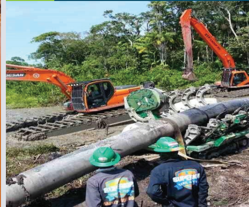
Fig.3a: Fusion/Installation of 22-inch HDPE pipe
