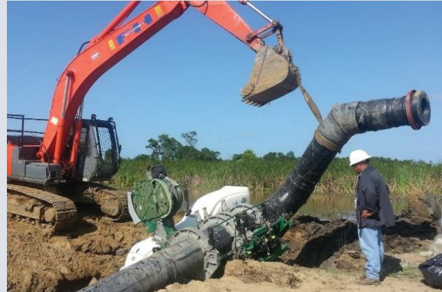
Fig.3: Fusion/Installation 22" inch HDPE pipe
